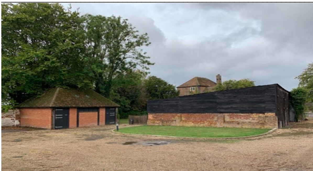
Figure 4: The storage barn (Building 3); Coldharbour House visible in background
